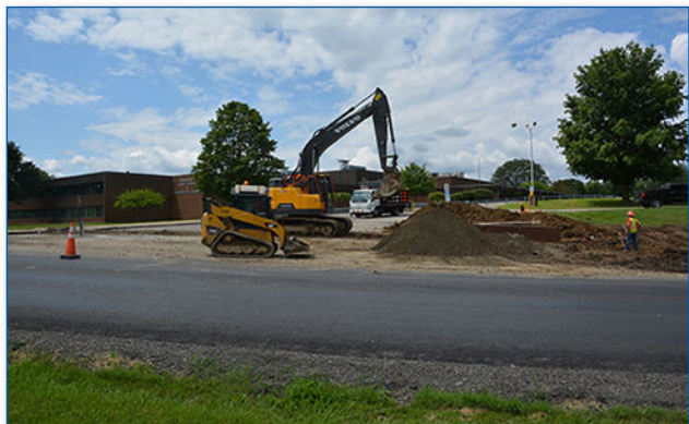
Construction on Sing Sing Road will widen the roadway.
